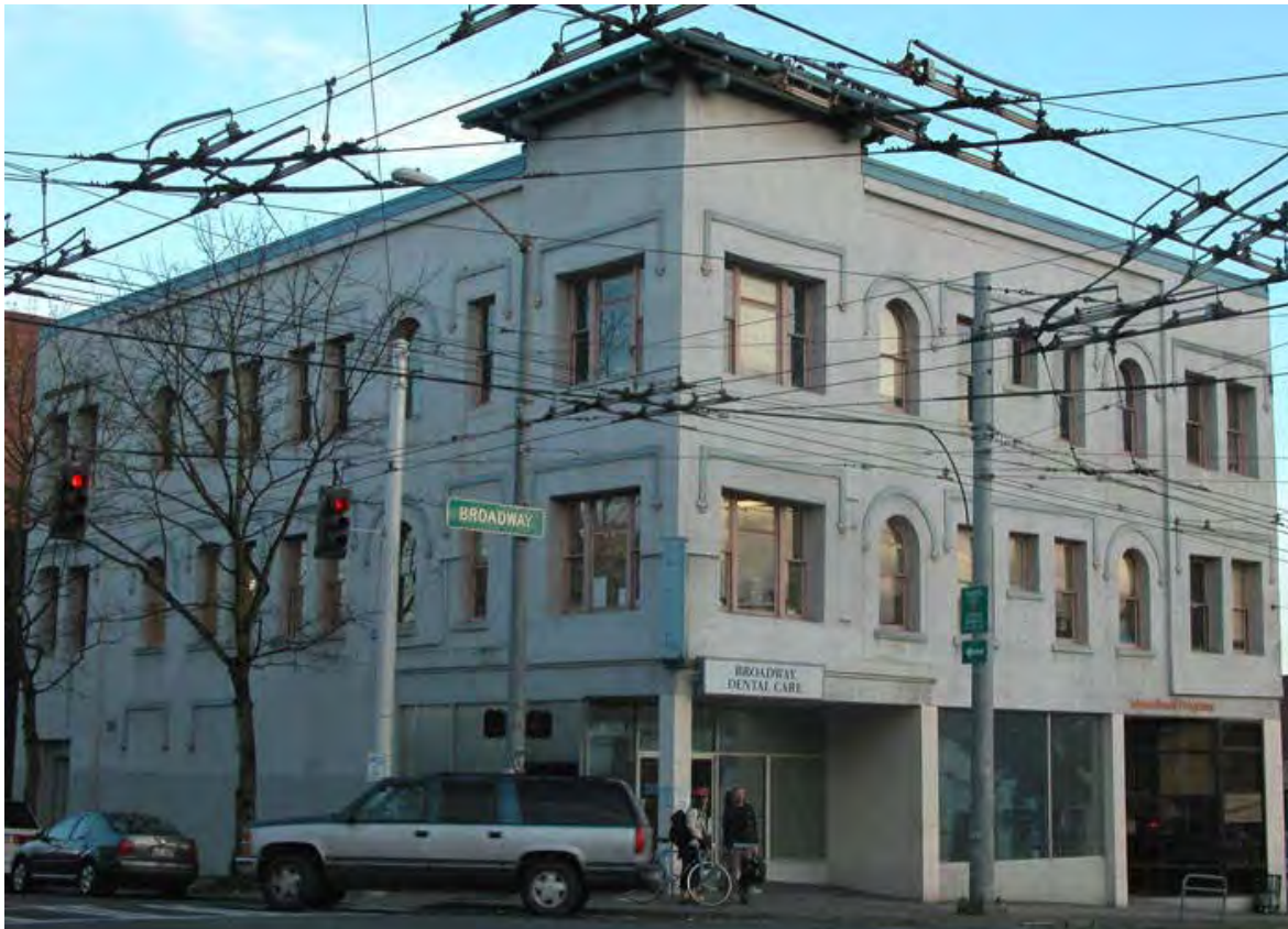
Fig 63 A 2006 view looking southeast at the north and west façades. (UW Libraries Special Collections, item no. 20060213AMB0049)
