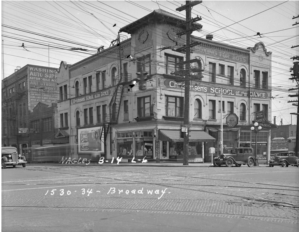
Fig 58 A 1937 view toward the primary west and north façades of the Booth Building, looking southeast from the intersection of Broadway and E. Pine Street. (King County Tax Assessor property record card, Puget Sound Regional Archives)
