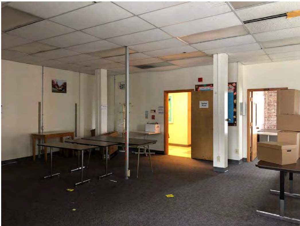
Fig 38 Typical upper floor classroom space, view looking back toward the corridor.
