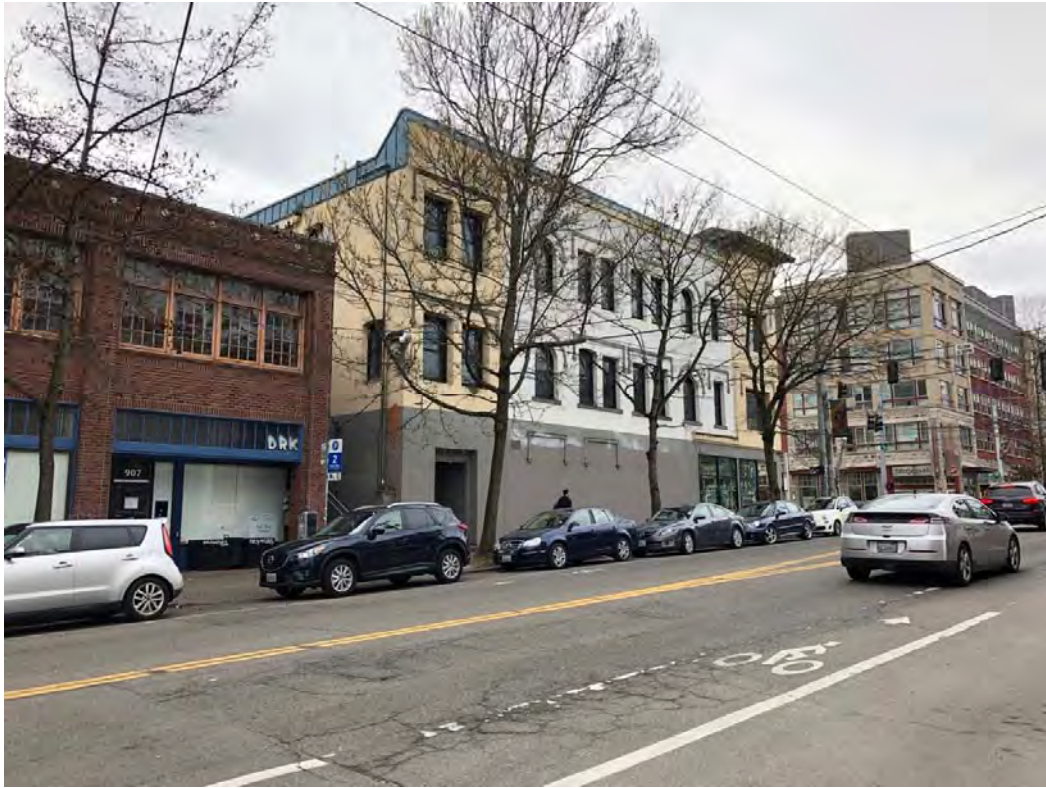
Fig 18 View southwest across E. Pine Street, toward the north façade and a portion of the east side.
