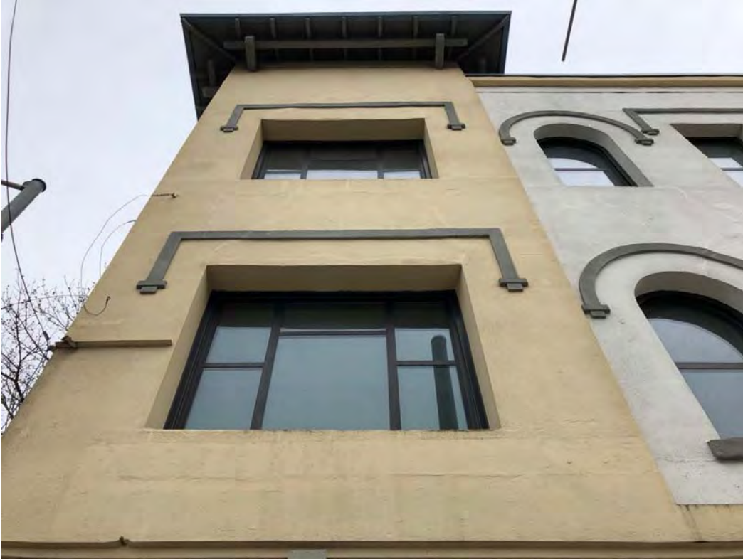
Fig 22 Detail view looking up at the north end of the primary west façade.
