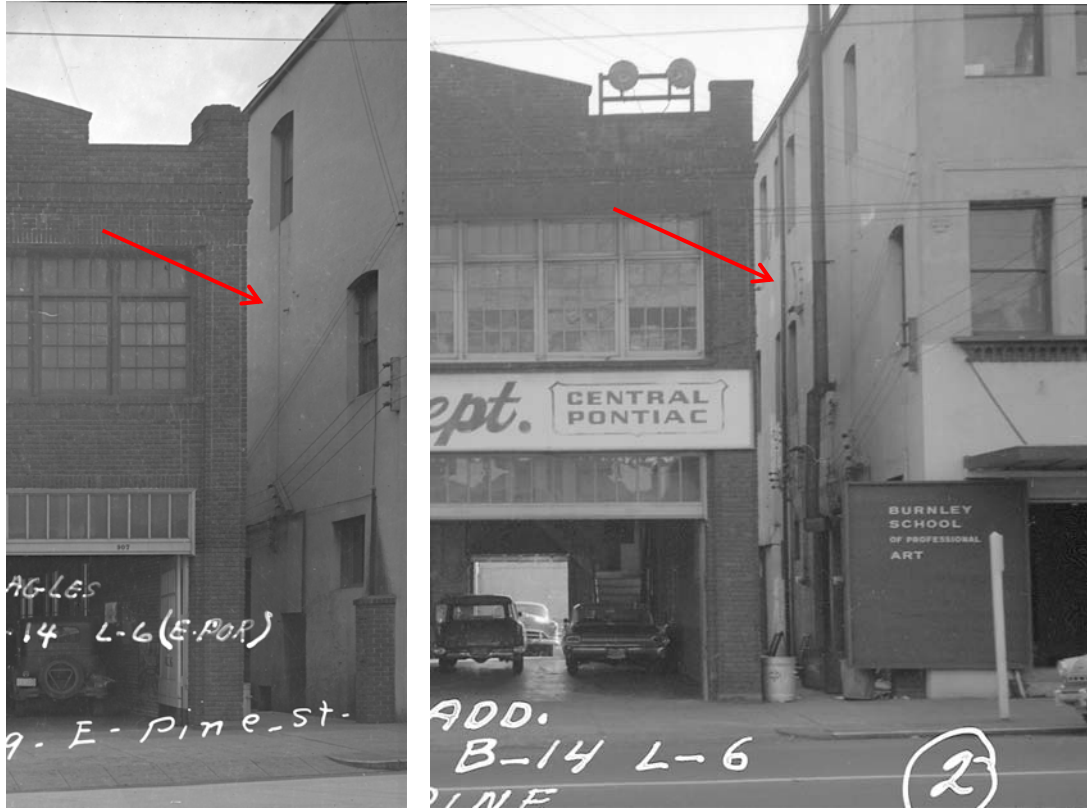
Figs 59 & 60 These 1937 and 1959 views from the property record card of the building at 909 E. Pine show a portion of the east and north sides of the subject building. (Puget Sound Regional Archives)
