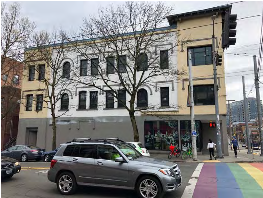
Fig 19 View south across E. Pine Street at the primary north façade.
