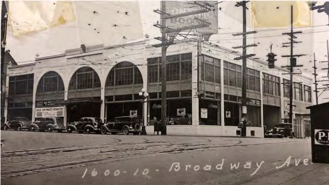
Fig 53 The former Boone & Company Pontiac dealership, at the northeast corner of Broadway and E. Pine, shown in a 1937 tax record photo. (Puget Sound Regional Archives)
