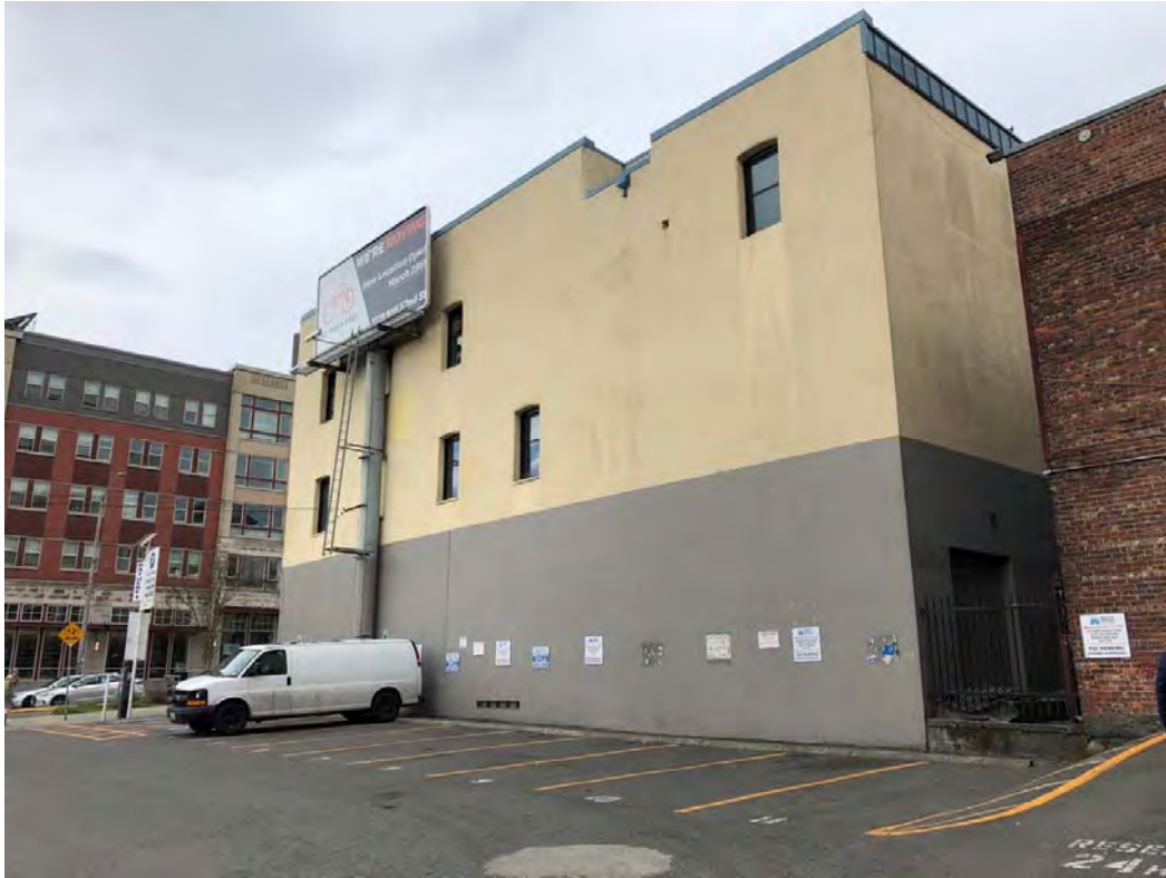
Fig 26 View northwest toward the south façade and the southern portion of the east side.
