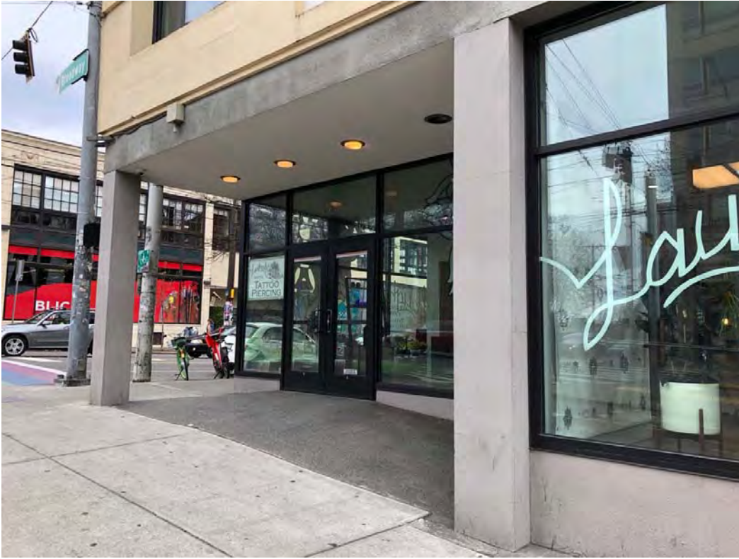
Fig 24 View northeast from the Broadway sidewalk, showing a portion of the central storefront and the recessed northernmost storefront.
