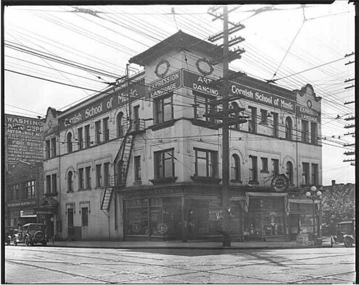
Fig 56 Above, view of the Booth Building ca. 1920, looking southeast from the intersection of E. Pine Street and Broadway. (MOHAL, item no. 1983.10.2175)
