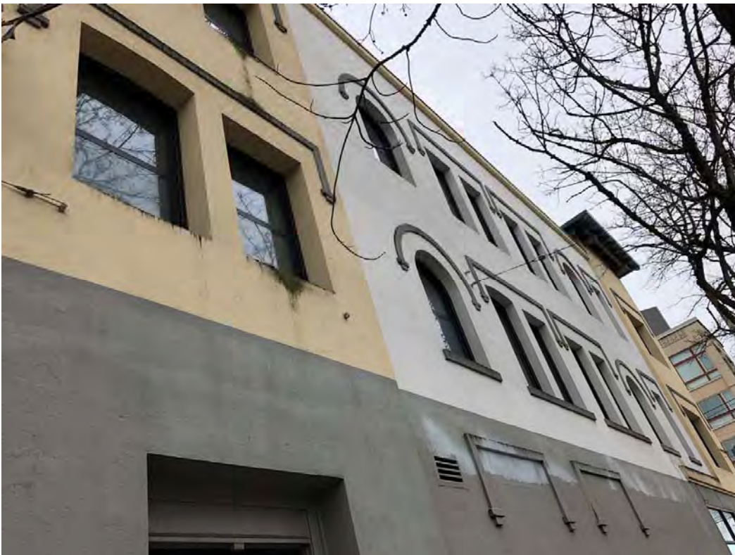
Fig 23 Detail view looking up along the north façade.
