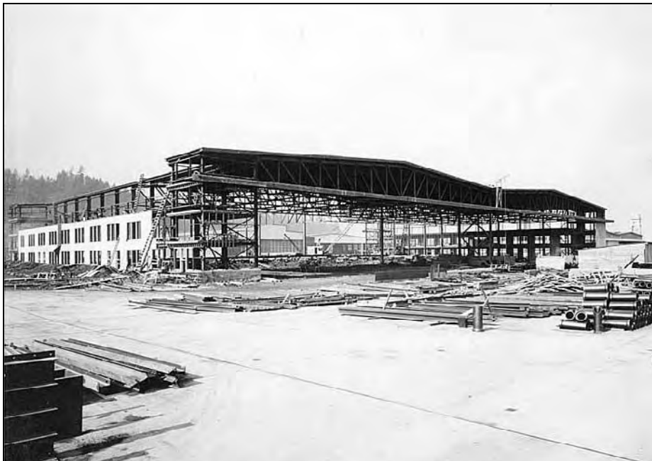
Construction of land plane hangar looking west showing south and east elevations. Photo Source: University of Washington Special Collections, Image No. SEA2803.
