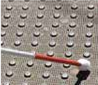
PRE-WEATHERED CAST IRON NATURAL IRON PATINA CAST-IN-PLACE, NON-SLIP Supplier: TUFTILE
