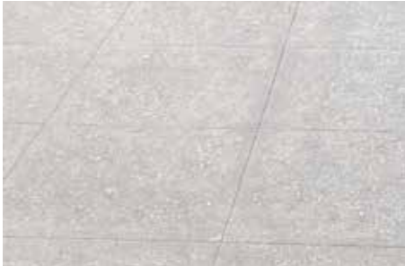
LIGHT GREY (LG) = SOLOMON ONYX 920 OR SIMILAR APPLIED AT 1% LOADING BROOM SWEEP SURFACE FINISH TOOLED 2'X2' JOINTS WITH NO SHINER
