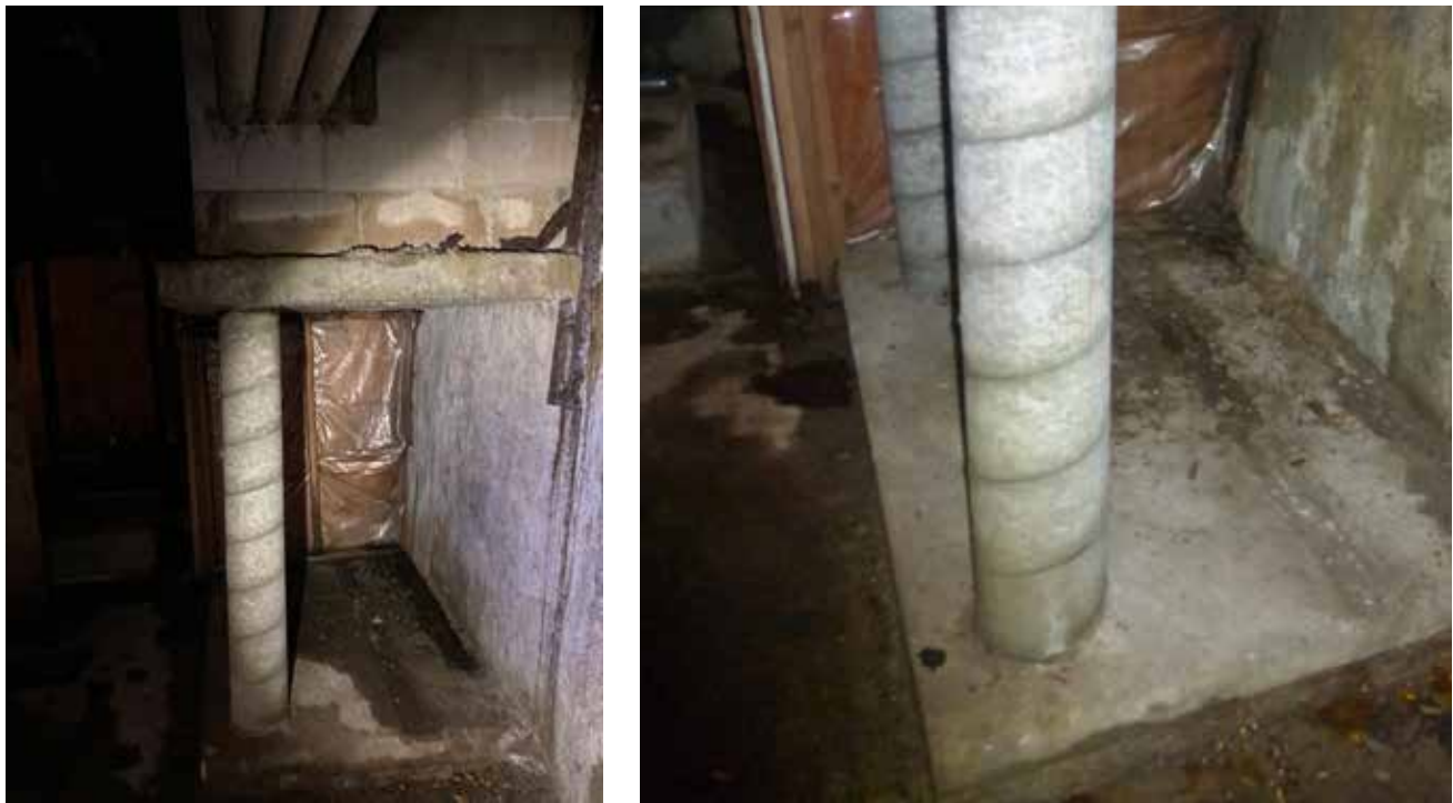
EXAMPLE OF CONCRETE COLUMNS AWAY FROM STREET WALL SUPPORTING AN ELECTRIC VAULT. Located in areaway 1603 at 3rd & Washington, SW corner in Pioneer Square.
