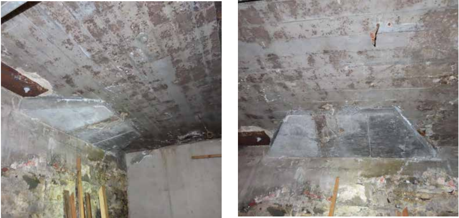
EXAMPLE OF CONCRETE SLAB UNDER RAMP (PROPOSED RAMPS ARE LONGER THAN SHOWN). Located in areaway A1301 at 1st & Washington, SE corner in Pioneer Square.
