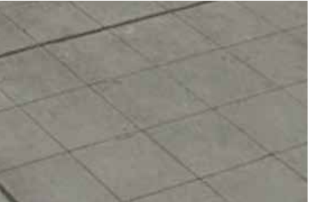
DARK GREY (DG) = SOLOMON SGS ONYX 920 OR SIMILAR APPLIED AT 4% LOADING BROOM SWEEP SURFACE FINISH TOOLED 2'X2' JOINTS WITH NO SHINER
