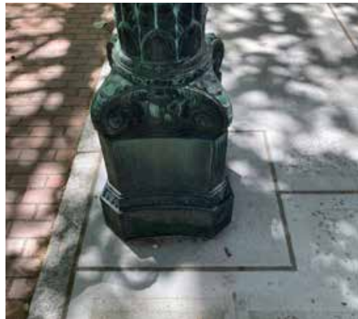
NEW CONCRETE OVER AREAWAY EXAMPLE AT OCCIDENTAL AND KING
