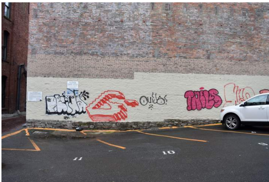
10 - This is the south west corner of the Bread of Life Mission building across the parking lot.
