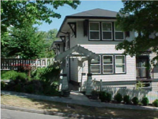
*Broad roof eaves improve aesthetics, reduce thermal gain in summer and divert rain away from foundation.*
