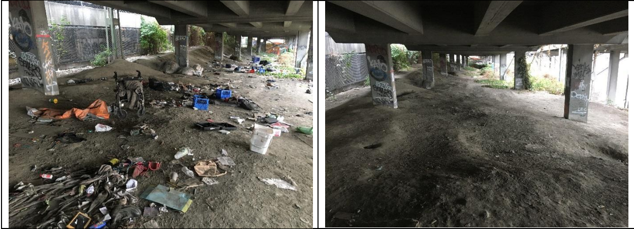
Above: before and after the cleanup under the Viaduct near Lenora Street
