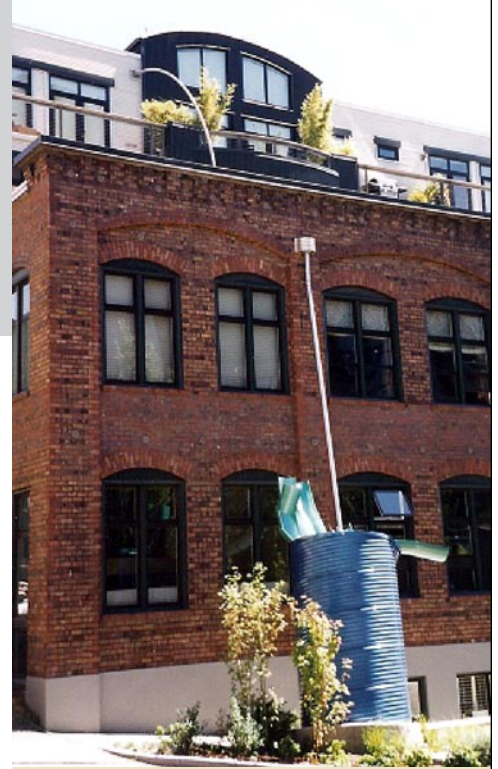
The Beckoning Hand Rainwater Cistern on Vine Street, Seattle, WA. Image courtesy of Mayfly Engineering and Design.
