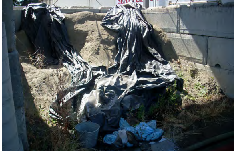
Current Material Storage is open, causing contamination issues
