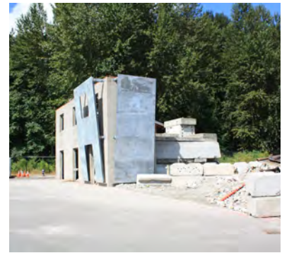
Existing Structural Collapse Prop
