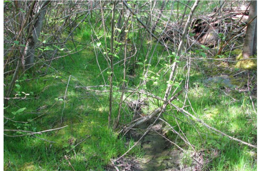
Photo 10 Roadside channel routing run-off to stormwater infiltration facility in PSE powerline right-of-way.
