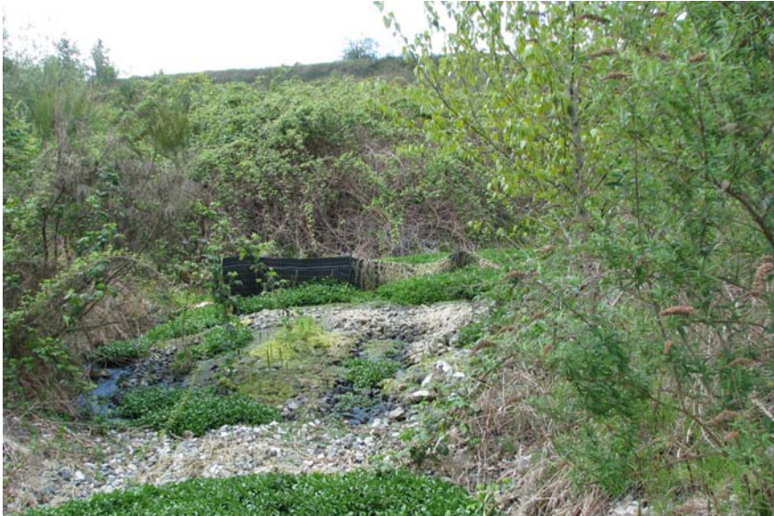
Photo 9 Stormwater conveyance ditch in the northeast portion of parcel B.
