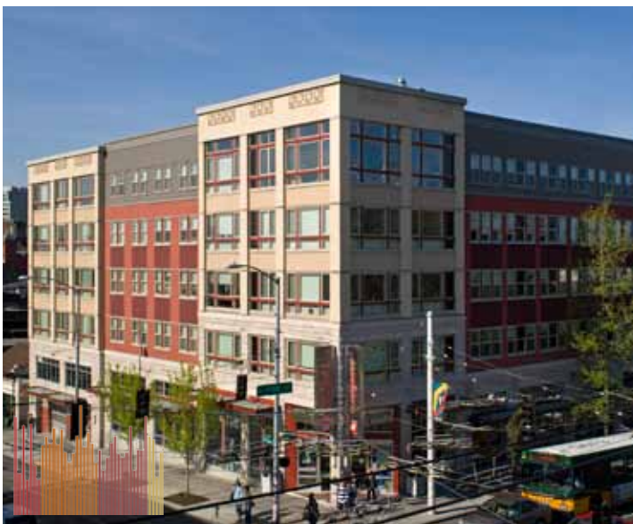
GGLO collaborated with Capitol Hill Housing to design Broadway Crossing (LEED Silver), and measure the building's performance after building occupancy. Lessons learned allowed the team to fine tune building operations. (Photo: William P. Wright)
