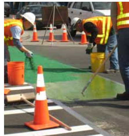
Installing a Green Bicycle Lane (Photo: Seattle Dept. of Transportation)
