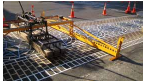
Creative crosswalk pilot project using DuraTherm heat-transfer plastic. (Photo: Seattle Dept. of Transportation)
