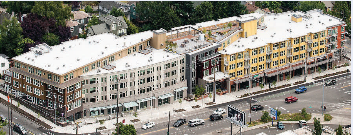
Prescott Wallingford Apartments: Jay Dotson Photography courtesy of TIAA-CREF
