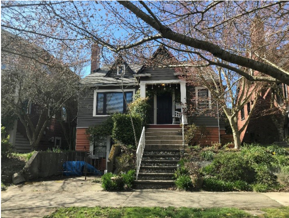
Typical Existing House in Seattle
