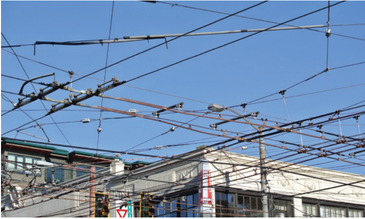
First Hill Streetcar: Overhead Electrical Work
