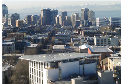
Looking over the top of the Bullitt Center
