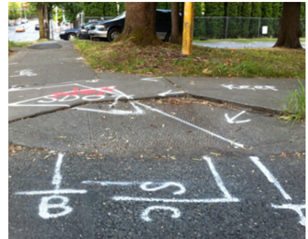
Broken Seattle sidewalk in the Central District
