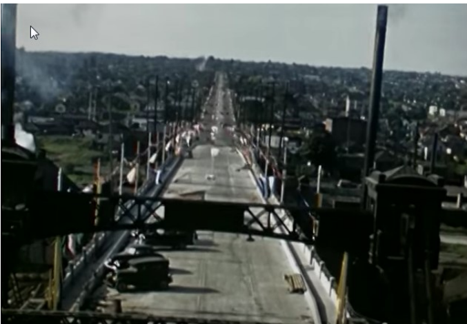
Construction and opening of the Ballard Bridge, 1940 Item 524 , Record Series 2613-09 , Seattle Municipal Archives
