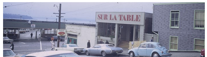
Sur la Table and Stewart House (l to r) on Stewart Street, October 1972. Item 33902, Seattle Municipal Archives
