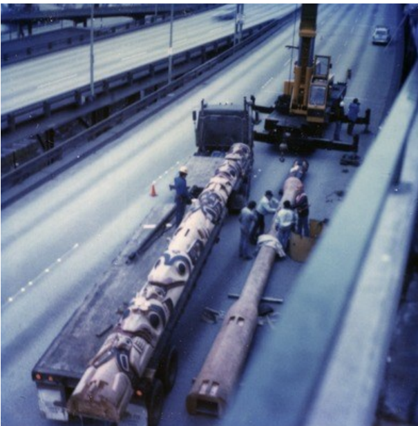
Totem pole #2 unloaded from truck on viaduct, 1984. Item 175588 , Seattle Municipal Archives
