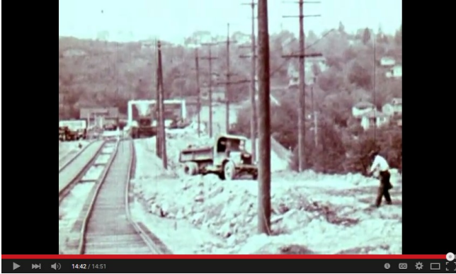
Spokane Street construction, 1928 Item 434 , Seattle Municipal Archives
