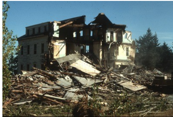
Discovery Park, Demolition of 423 Building, September 30, 1987 Item 170416, Seattle Municipal Archives
