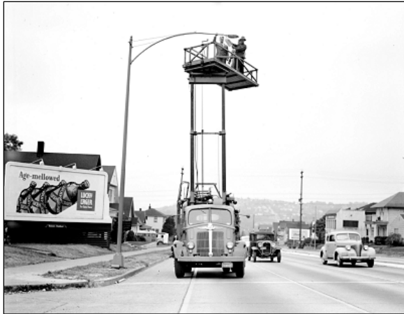
Tower truck in operation, August 10, 1949. Item No. 41894, Seattle Municipal Archives
