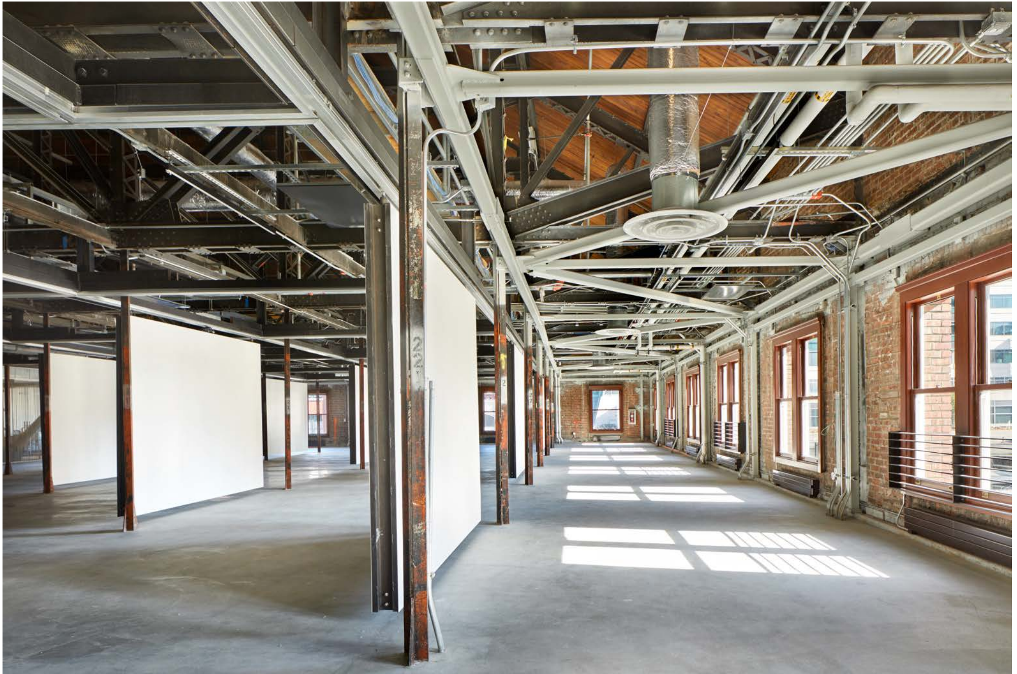
ARTS at King Street Station | Cultural Space with sample gallery wall configuration | Photography by Benjamin Benschneider
