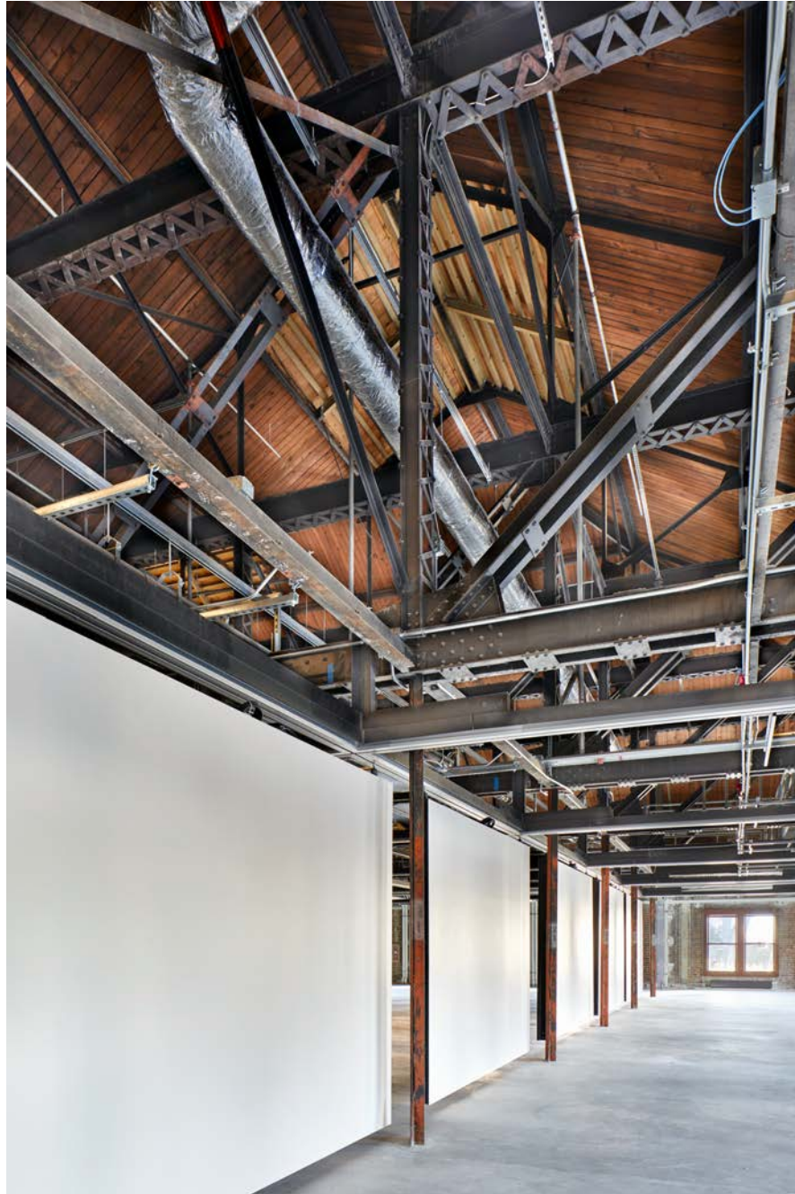
ARTS at King Street Station | Cultural Space, view of high ceiling | Photography by Benjamin Benschneider
