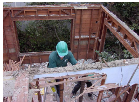
Worker salvaging reusable dimensional lumber during a home deconstruction.
