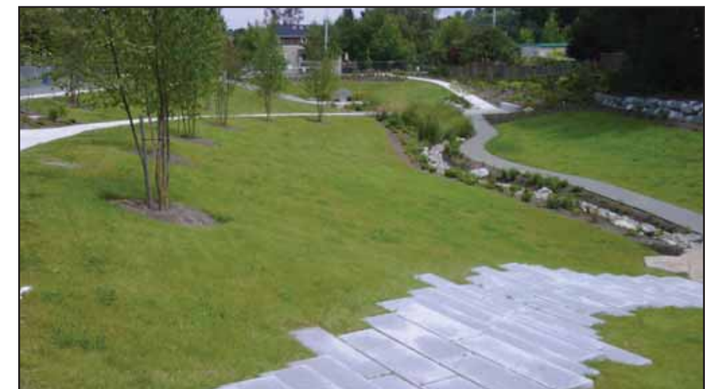
Phase 1 above-ground stormwater storage facility
