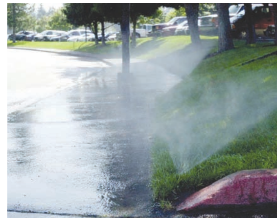
Example of a wasteful irrigation system.
