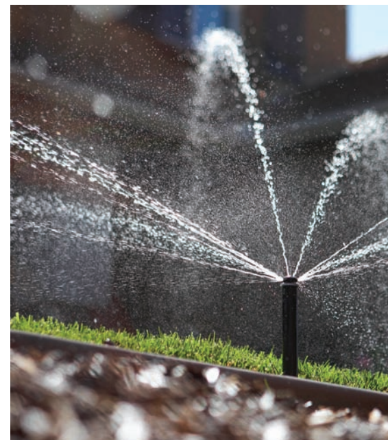
Efficient sprinkler heads provide water more slowly, rotate to provide water more evenly, and operate without overspray.
