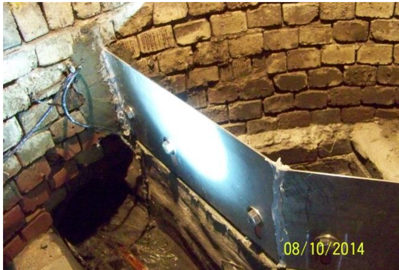
Figure 4-6. Outfall 30 Raised Weir Installation
