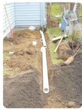
DOWNSPOUT TO RAIN GARDEN PIPED CONNECTION
