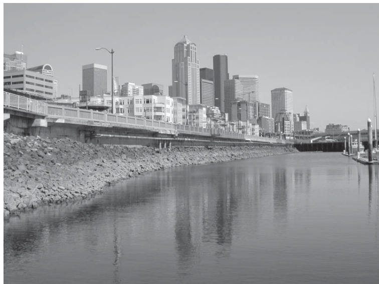
Rip-rap protecting the sea wall on Elliott Bay. Photo by Duncan Kelso
