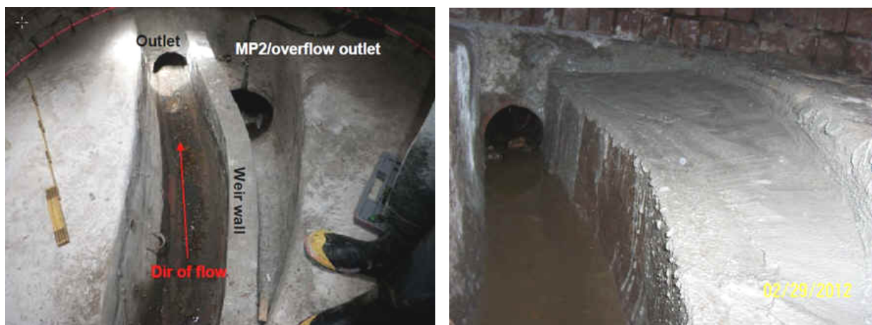
Figure 4-1. Before and After Seal-up at Overflow Structure 41A
