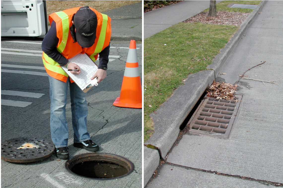
Figure 1. Round top (left) and grated (right) basins within the City of Seattle. Round top basins are normally situated within the roadway at one or more corners of intersections and receive stormwater through pipes from inlets (small catch basins) along nearby curbs. In contrast, grated basins are normally located along curbs and primarily receive stormwater directly from the road surface.
