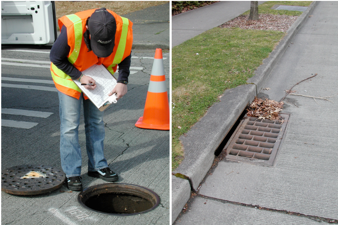
Figure 1. Round top (left) and grated (right) basins within the City of Seattle. Round top basins are normally situated within the roadway at one or more corners of intersections and receive stormwater through pipes from inlets (small catch basins) along nearby curbs. In contrast, grated basins are normally located along curbs and receive stormwater directly from the road surface.
