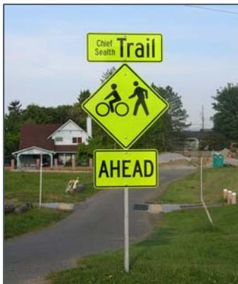
Figure H-3. Advanced Warning Sign Subplates
