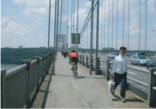
George Washington Bridge, NYC
