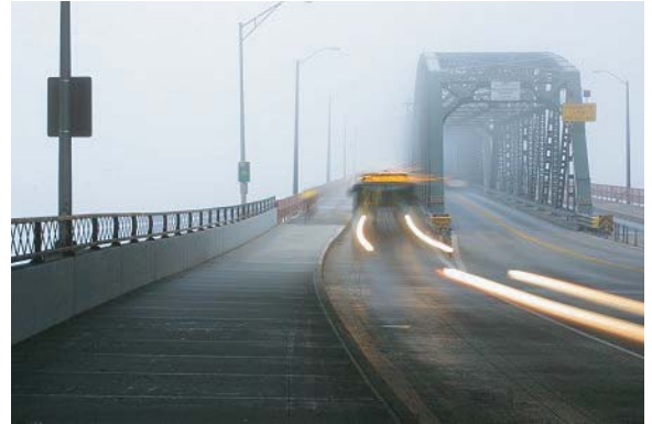
Hawthorne Bridge, Portland
