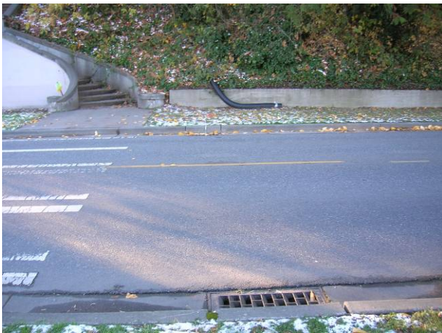
Figure 4. Outfall to temporary pipe on west side of roadway
