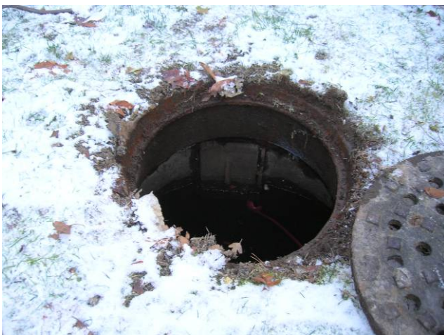
Figure 5. Outlet to upstream manhole
