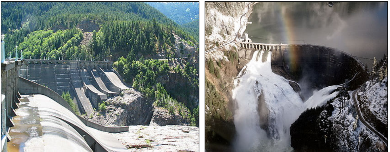
Figures 5 and 6. Diablo spillways under normal conditions and in use.
