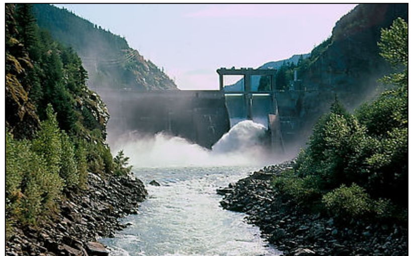
Figure 10. Gorge Dam spilling.
