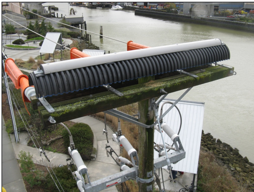
Figure 6-2. Osprey nest excluder and insulated conductor covers.
