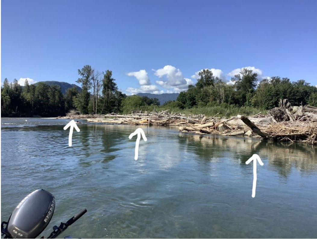
Figure 5.6-25. Looking downstream at PRM 72.1. Right arrow is dolotimber revetment structure along roadside bank, center arrow is dolotimber apex jam, and left arrow is natural apex jam at PRM 72.0. Large wood Tag ID 65 is in the central dolotimber apex jam. Large wood Tag ID 67 is in the natural apex jam on the left. Photo is taken August 5, 2021.
