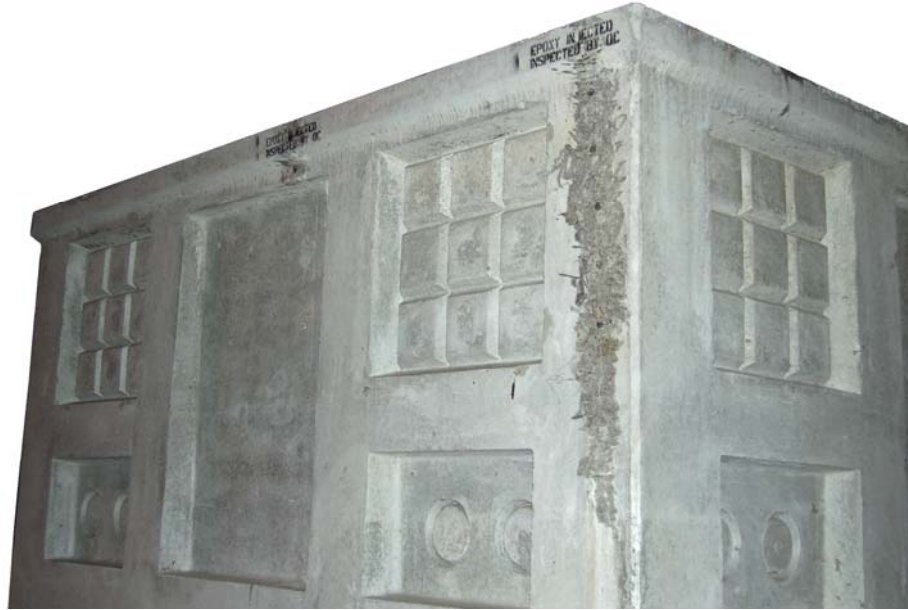
Figure 1. Vault Repaired with Epoxy Injection
