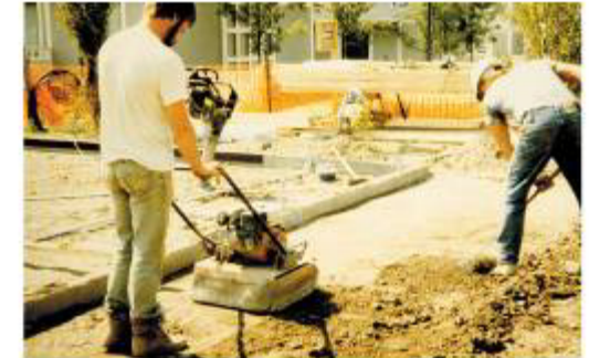
Fig. 1.2 Compaction is necessary to create a load-bearing surface on which to lay pavement.
