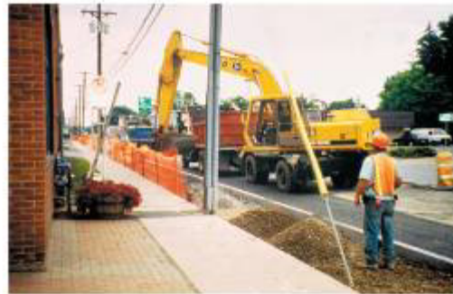
Fig. 1.9 Installing CU-Structural Soil™ in Ithaca, NY in 1997
