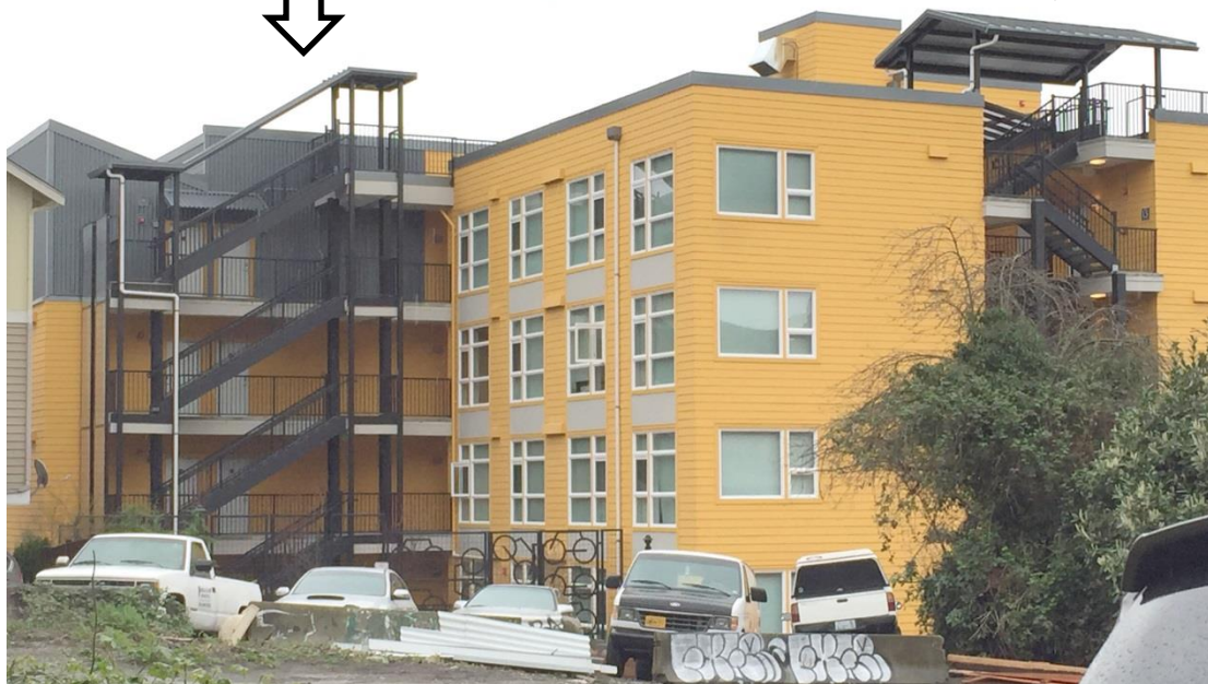
Back of building.
