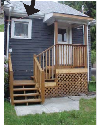
After: safe, sturdy construction with treated wood and handrails
