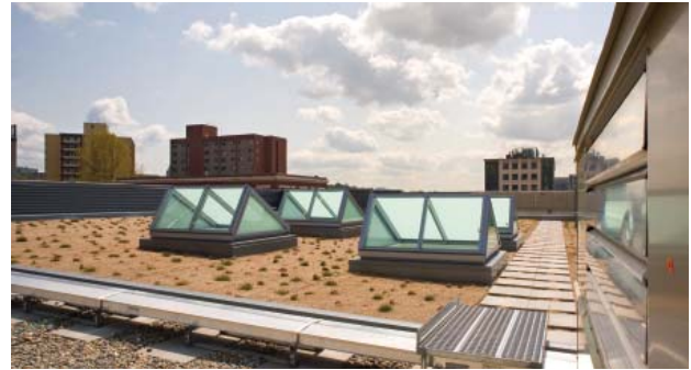
Green roof. Photo by Michael Burns.
