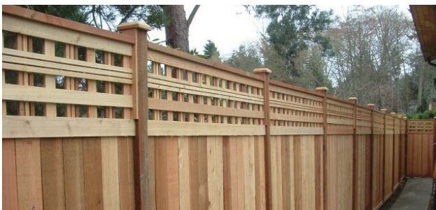
Fences do not count toward lot coverage and are also allowed anywhere on your property.
