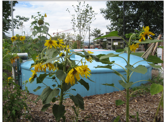
The Cascade People's Center uses rainwater collected from the roof and stores it in a cistern for toilet flushing.
