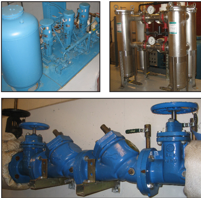
Pumps, filters and backflow prevention, King Street Station, Seattle, Wash. Images courtesy of Mayfly Engineering and Design, PLLC.
