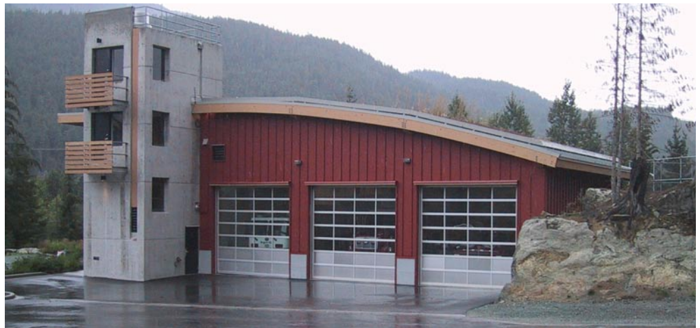
Spring Creek Fire Hall exterior (Courtesy of Stantec)
