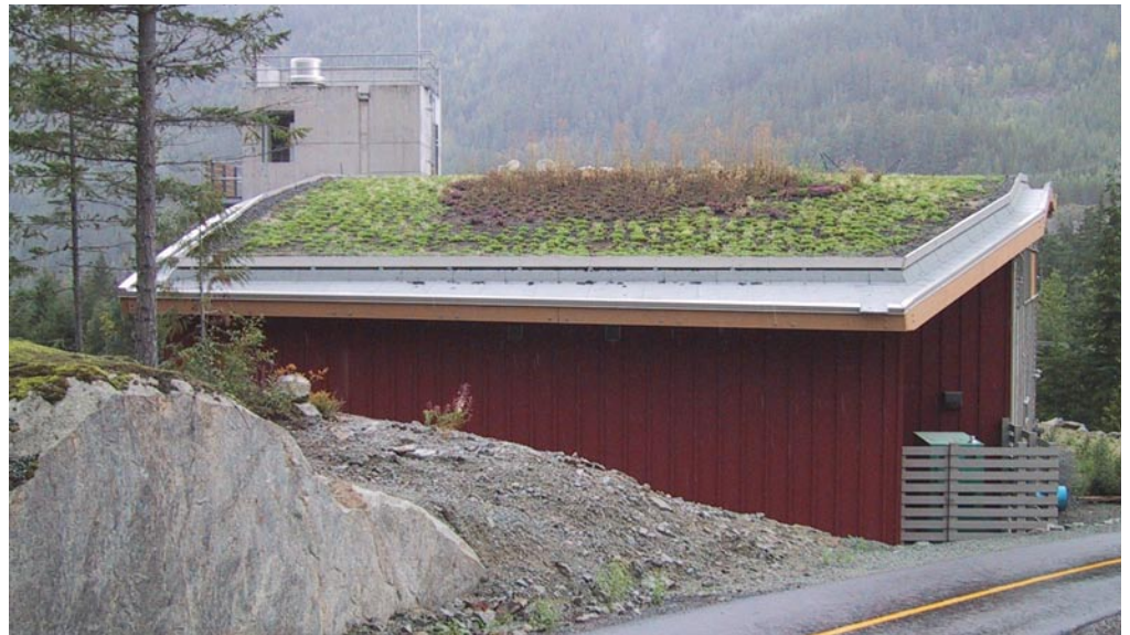
Spring Creek Fire Hall green roof & Valley Trail (Courtesy of Stantec)
