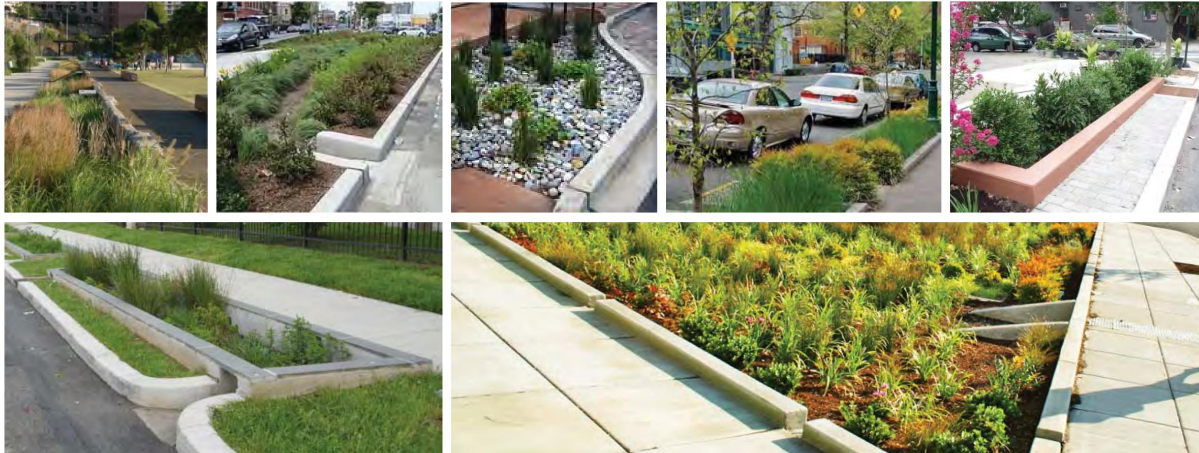
Through the process of **bioretention**, sediments and contaminants are removed from stormwater using Green Stormwater Infrastructure (GSI) practices such as bioretention ponds, rain gardens and bioswales.
