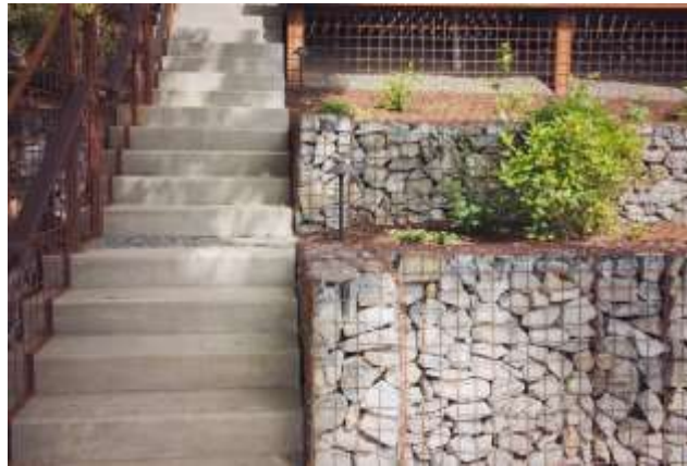
Example of Gabion Wall Regensis Ecological Design Landscape Contractors
