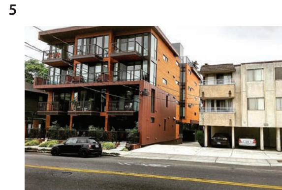
TERRACED OUTDOOR DECKS @ NEARBY APARTMENT
