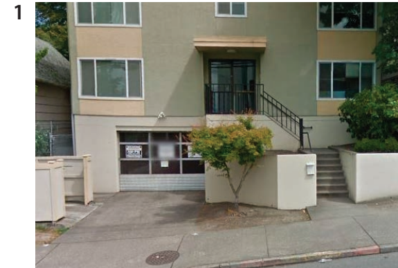
1 STEPPED, STREET-FACING ENTRIES
