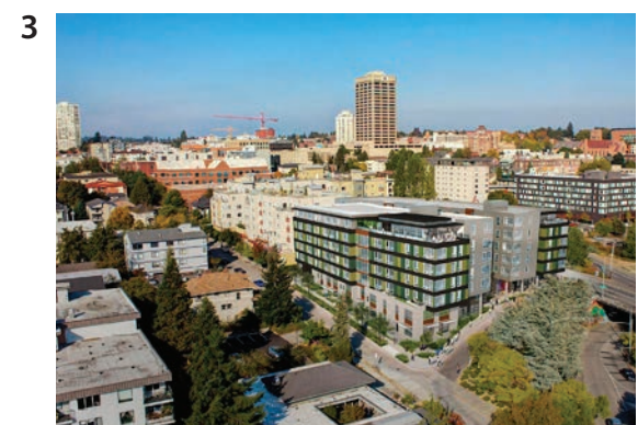
NEWLY-BUILT DENSE DEVELOPMENT TO SOUTH
