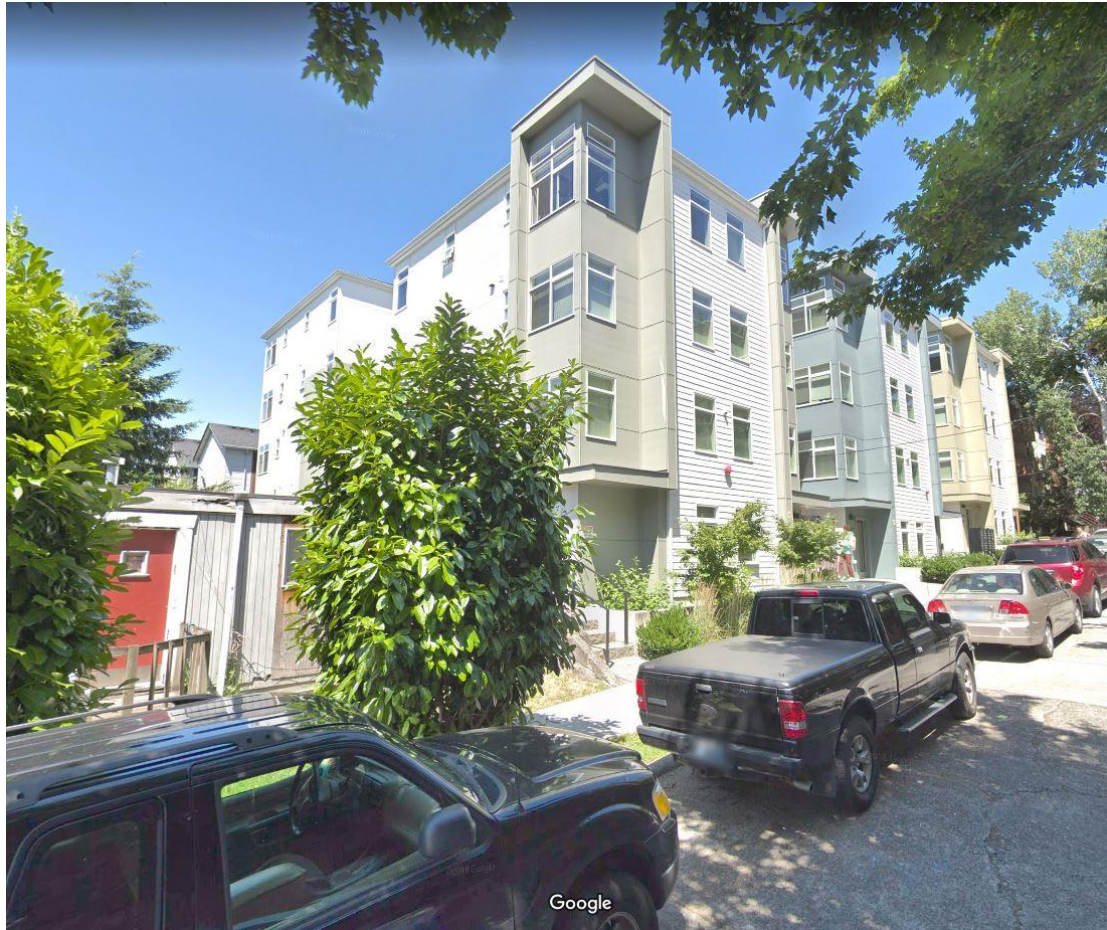
Neighboring Building to North
