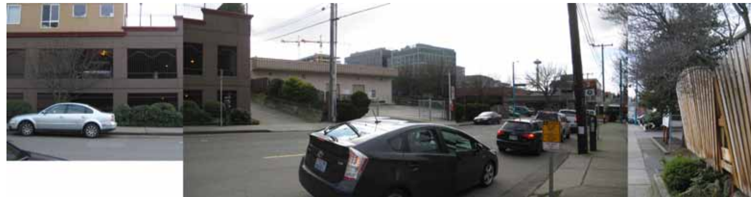
3 Northeast corner view of 400 Fairview
