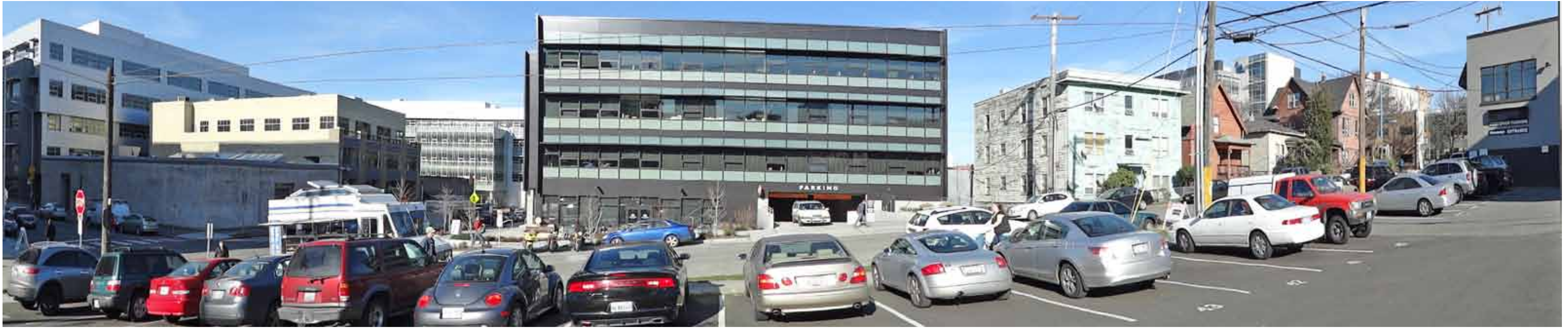
VIEW NORTH TO SITE - ALONG REPUBLICAN ST.
