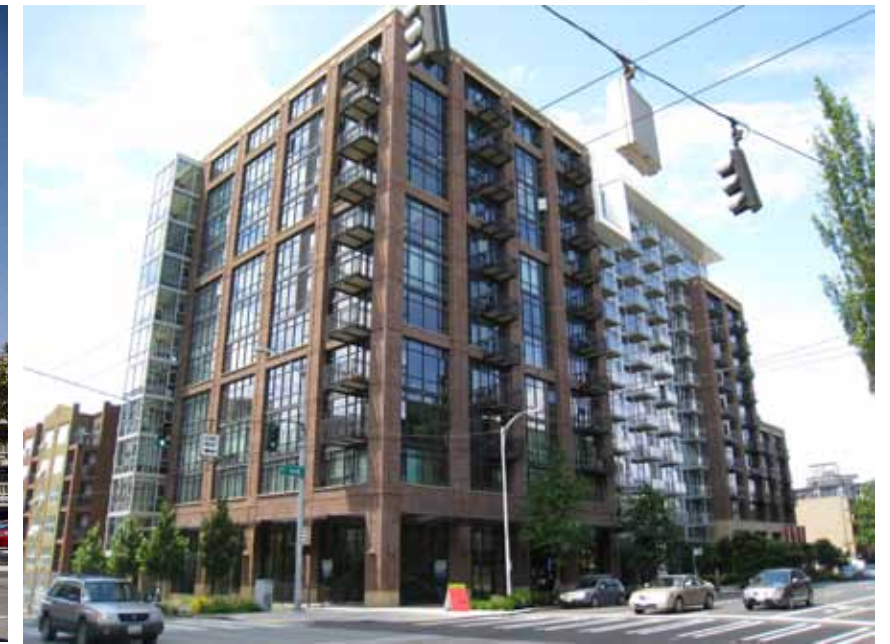
Large expanses of glazing for residential units.
