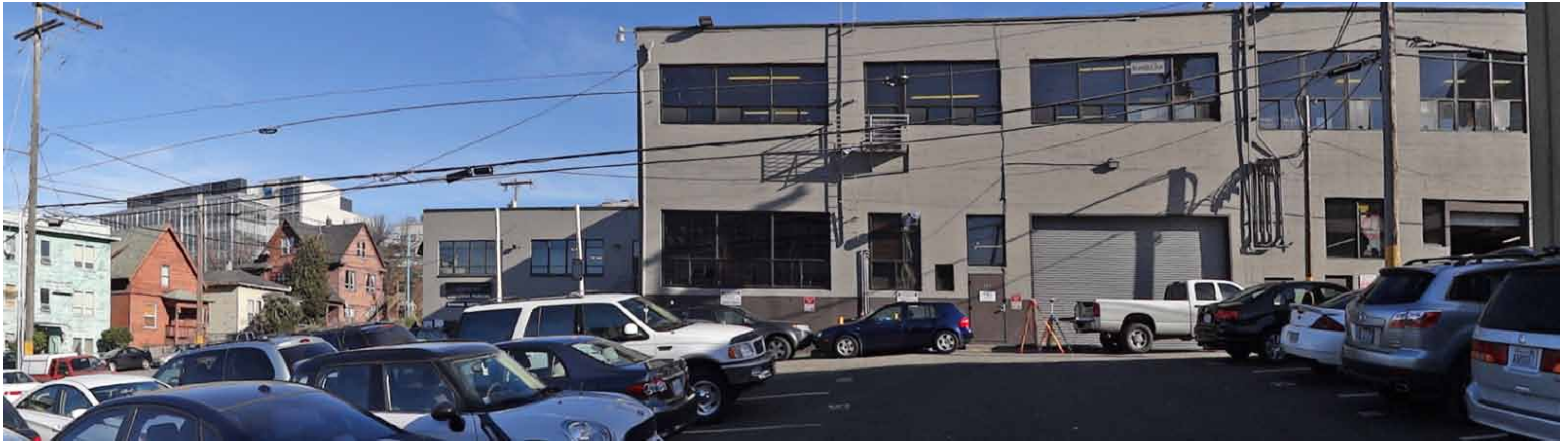
VIEW EAST TO SITE - ALONG ALLEY
