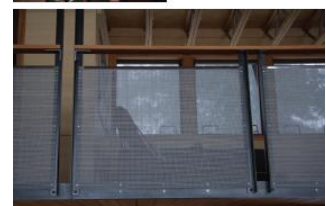
Metal sunshades and screens
