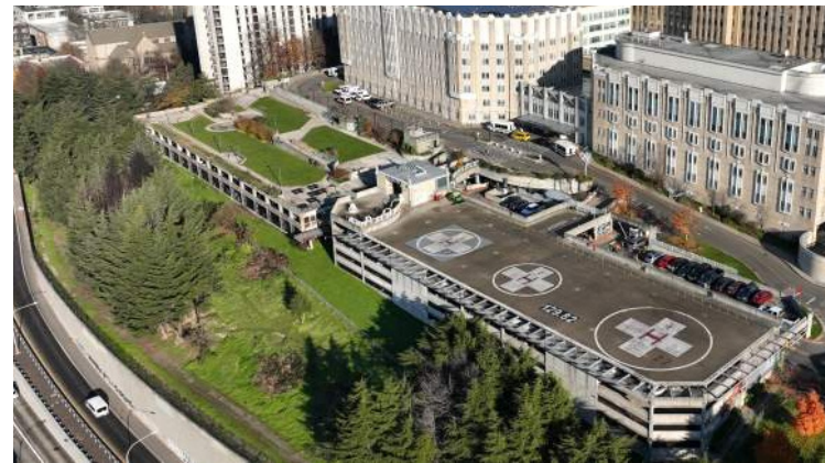
9 View Park Garage I & II 1974 - 2001
